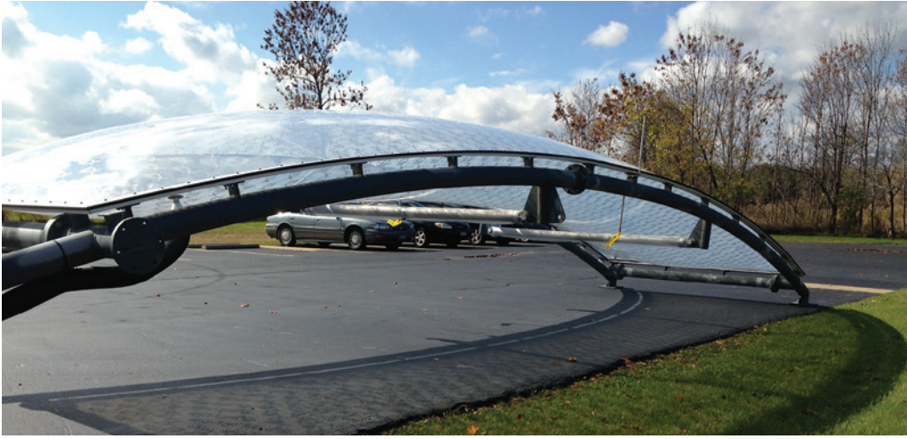
Here it is easy to see what kind of shading can be provided when utilizing some sort of print pattern on the ETFE film.
