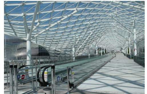
The above glass canopy at the exhibition fair in Milan, Italy, (by Architect Massimiliano Fuksas) is a masterpiece of engineering construction. However, due to the limited span capacity and the rigidity of glass, a very heavy steel structure with a triangulated configuration was required to achieve the organic shape.
