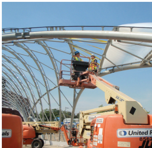
ETFE Cushion System being installed at Empire City's Casino, Yonkers, NY
