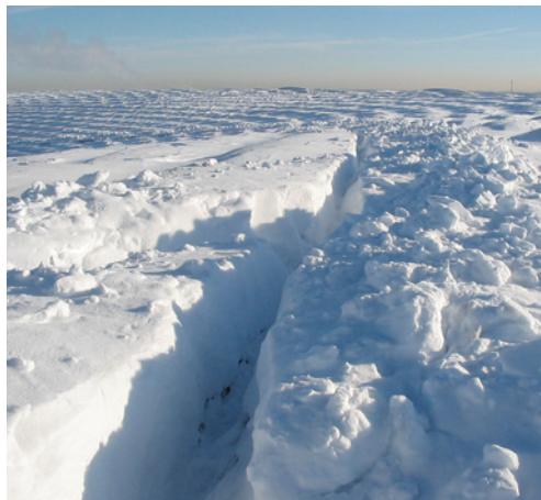
ETFE cushions under snow loads at the Allianz Arena, Munich, Germany
