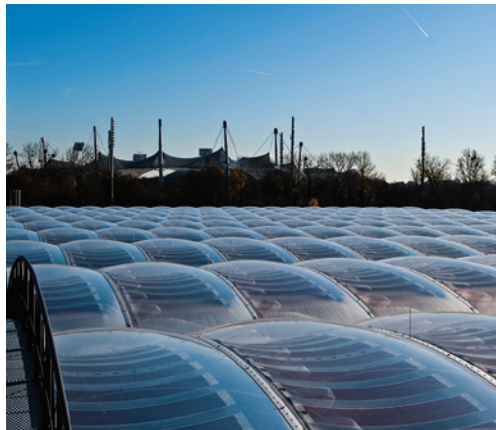
The roof of Munich's Municipal Waste Management Department
