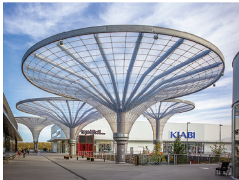
Here is an example of single layer pre-stressed structure and of an inflated structure.
