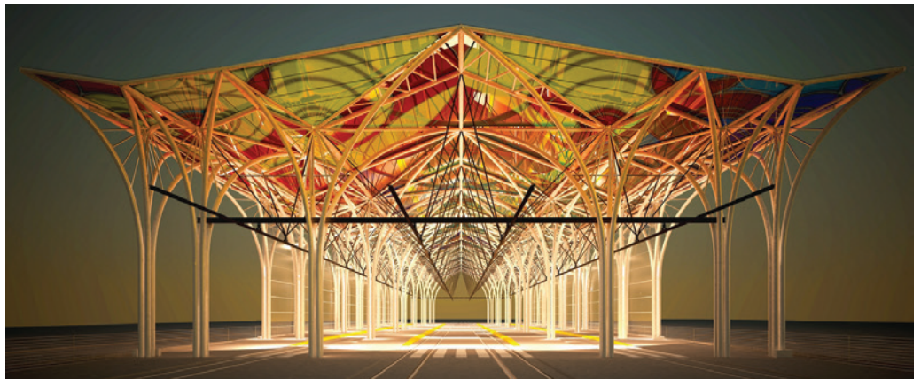
This picture shows the latest development in ETFE printing. With new digital technology, it is now possible to nearly print anything on the ETFE.
