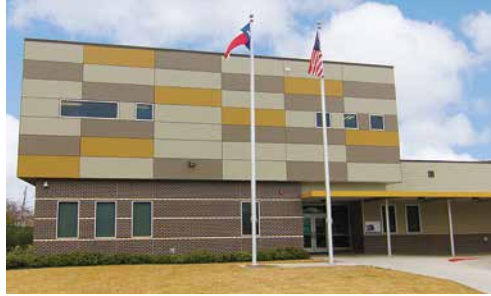
Extruded aluminum trim painted black accents the reveals in the façade to bring variation to the fiber cement panel.
