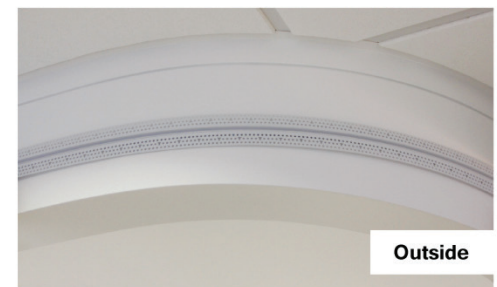
The flexibility of vinyl reveals also allows them to conform to curved walls and soffits. The minimum inside and outside radius is determined by the width and depth of the reveal, the 1/4" x 1/4" reveal being the most flexible.
