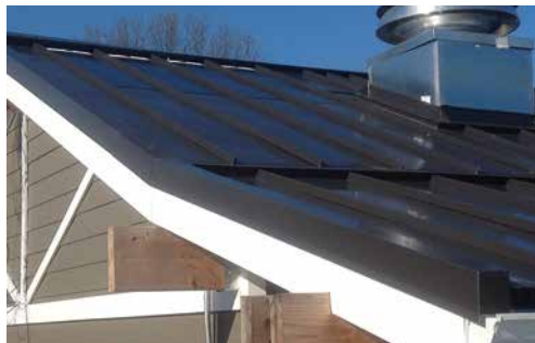
Figure 6 Metal roofs are ideal application for flexible peel and stick style solar power modules. Collection units can be custom made to fit between the metal panel seams without interfering with the visual look nor adding substantially in weight.
