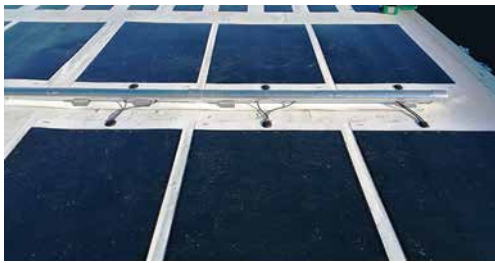
Figure 5 Unlike traditional rack mounted solar collectors, flat and flexible solar modules add very little weight to the roof.
