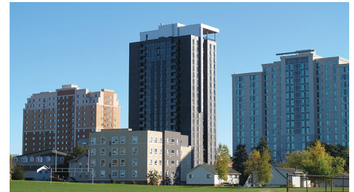
All the buildings in this photo are built using ICFs. Photo courtesy of Fox Blocks®
