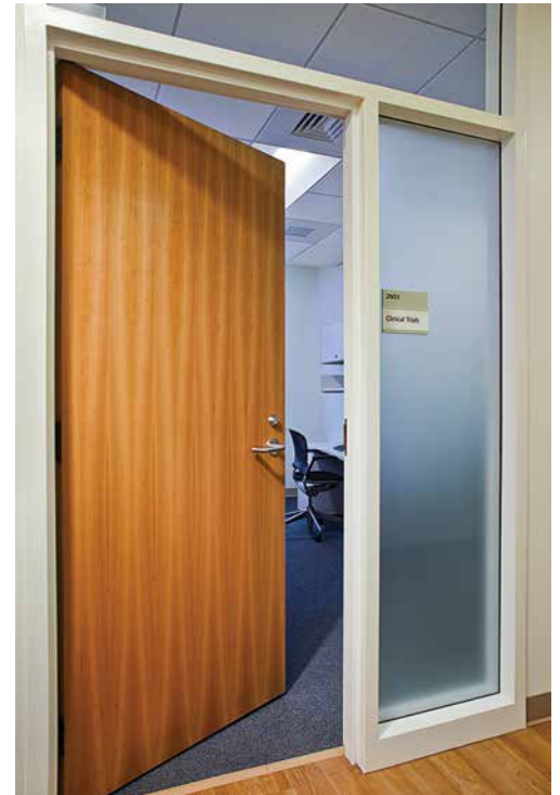
Finish options protect wood from moisture, handling damage, and harsh chemicals, and can be applied in either a factory or in the field under jobsite conditions.
